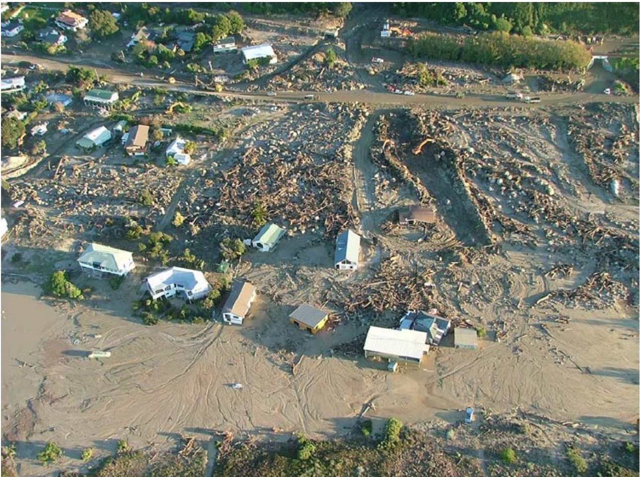
FIGURE 26: Debris Flow Damage, Awatarai Stream, Matata, New Zealand, following the 18 May 2005 debris flow event. McSaveney, et al (2005).
