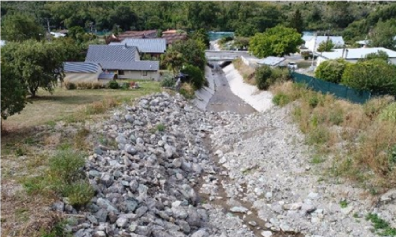
FIGURE 54: Rock and concrete lined conveyance channel, Roxburgh (Golder, 2019)
