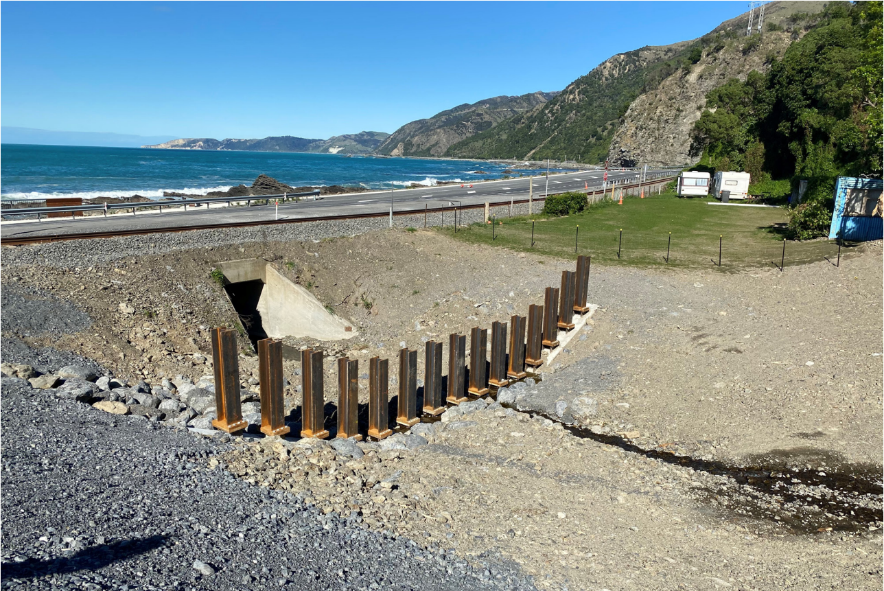
FIGURE 51: Debris Straining Structure, Rosy Morn Stream, Kaikoura Coast. Photo courtesy NCTIR
