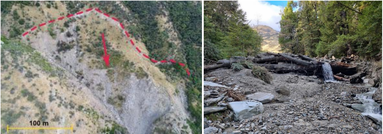
FIGURE 11: Left - Evidence of bank erosion and large-scale active slope instability of colluvium along a debris flow affected channel; Right - Partial deposition: Large boulder and woody debris deposits in the main channel of a steep creek.
