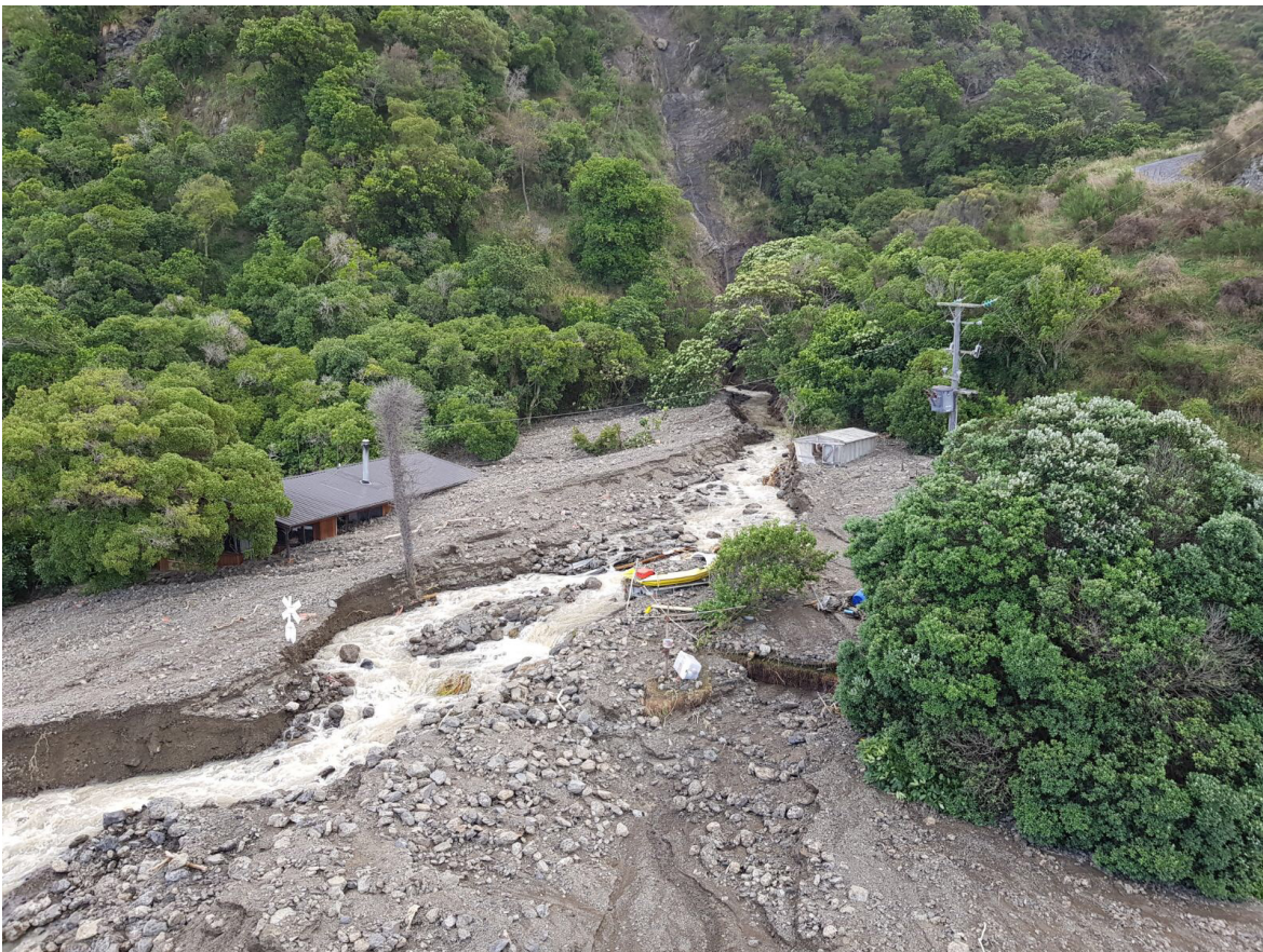
FIGURE 1. Debris flow impact on a timber framed house and inundation of road and rail (foreground) at Rosy Morn Stream, south of Kaikoura, following Cyclone Gita (February 2018). Photograph courtesy of NCTIR.
