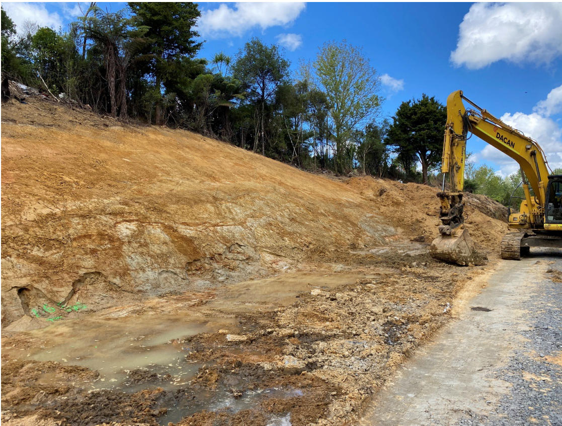
FIGURE 30: Temporary cut slope in a semi-intact block of residually weathered Pakiri Formation soil. Groundwater seepage is encountered at the toe in a silt-dominant soil layer, at or close to the basal failure surface of the block.
