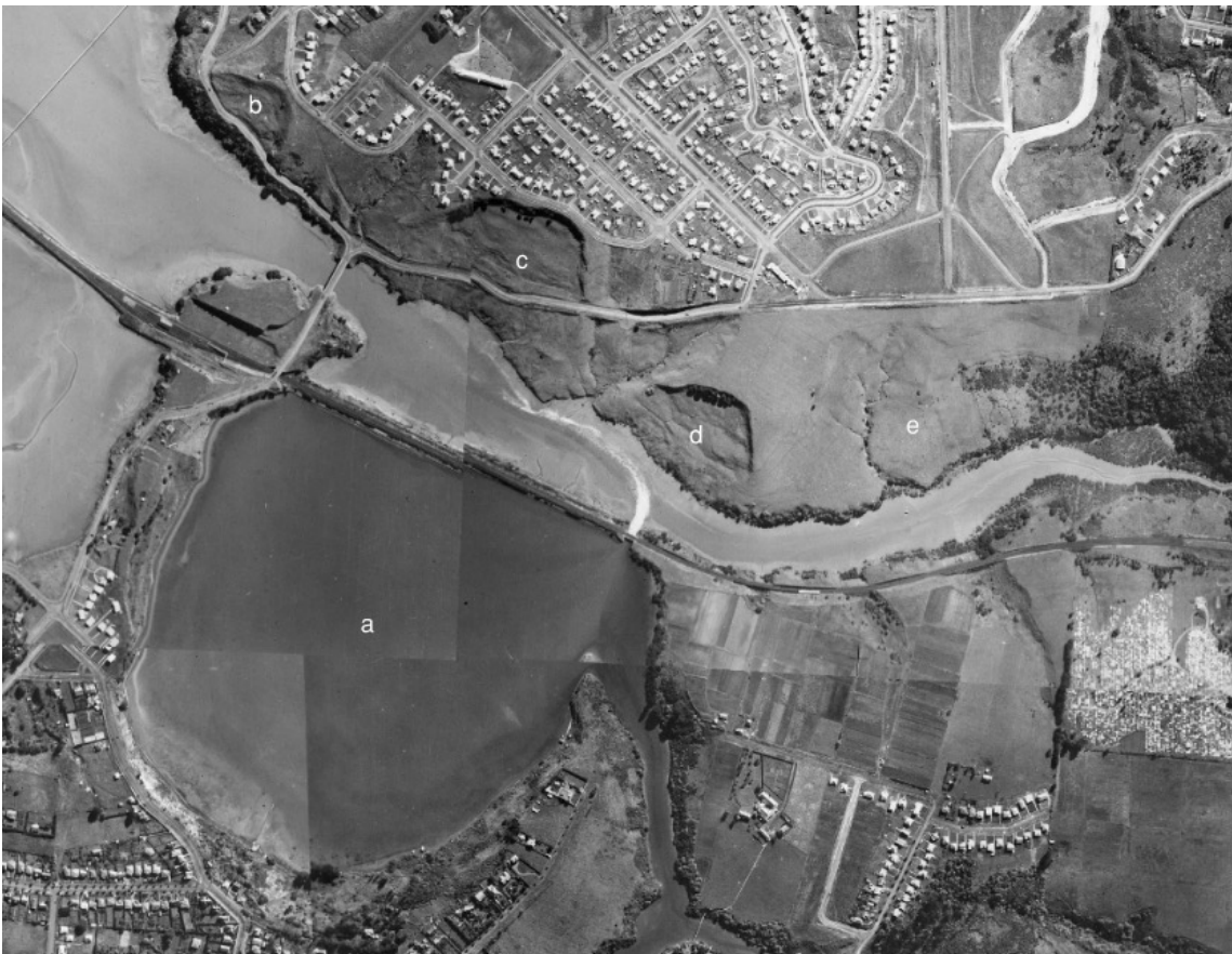
FIGURE 39: Orakei Basin and the landslides of the north-eastern flank, labelled as follows: a) Orakei Basin, b) Ngapipi Road Landslide, c) Kepa Road Landslide, d) St Josephs Landslide, e) Pourewa Landslide. Base imaged sourced from Auckland Council GeoMaps, 1940 aerial photograph layer.
