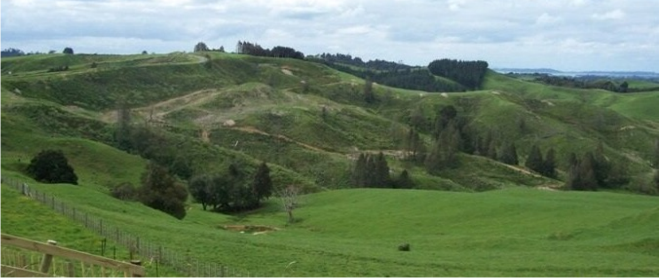
FIGURE 18: Deep seated block slide in the Southern Landslide Zone.
