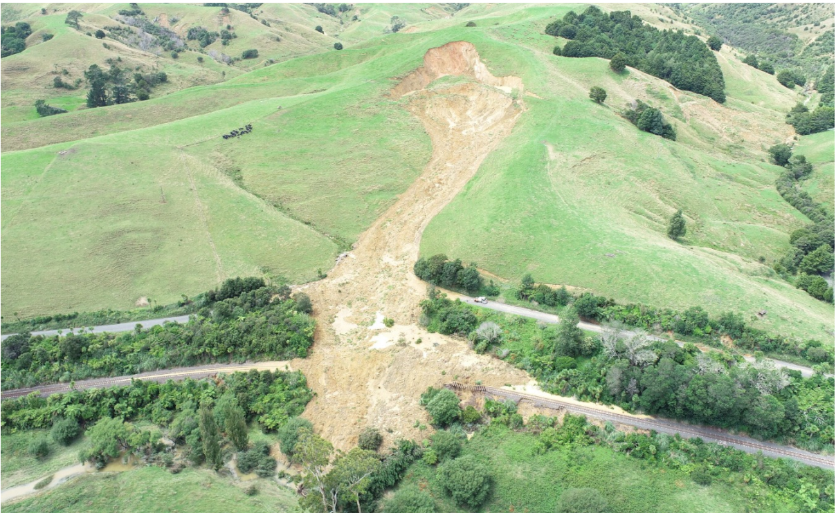
FIGURE 22: Rotational slide transitioning to debris flow in East Coast Bays Formation resulting in inundation of the road and railway line, with debris reaching the stream.
