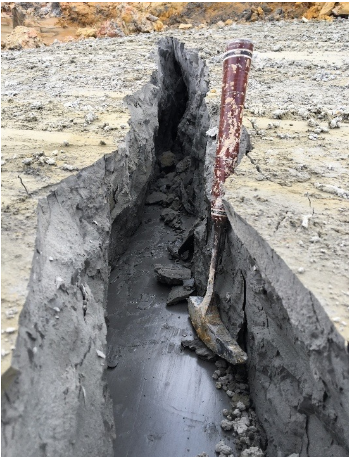
FIGURE 13: Shear plane at the contact between residual silt-dominant (upper) and clay-dominant (lower) soil layers of the East Coast Bays Formation .
