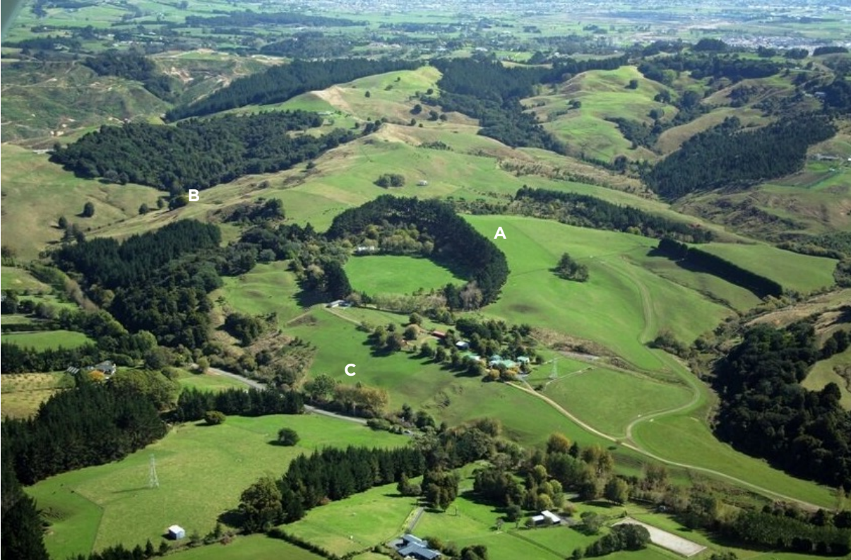
FIGURE 5: A tilted block of East Coast Bays Formation in the Southern Landslide Zone, demonstrating broad slopes parallel to bedding (A) and steep back-bedding geomorphology (B). Localised shallow-seated instability geomorphology is evident on the steeper slopes (C).
