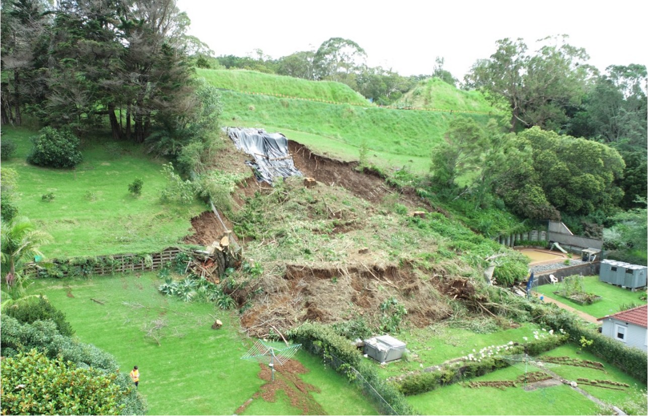
FIGURE 11: Rotational slide on the flank of Ōwairaka (Mount Albert) after heavy rainfall (2023).
