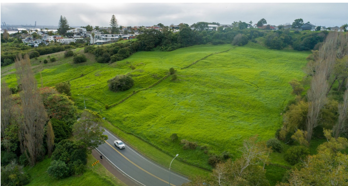
FIGURE 12: Keba Road landslide. See Section 5.1 for case study.
