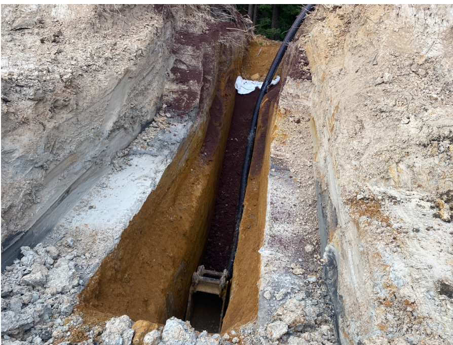
FIGURE 38: Counterfort drain installation.
