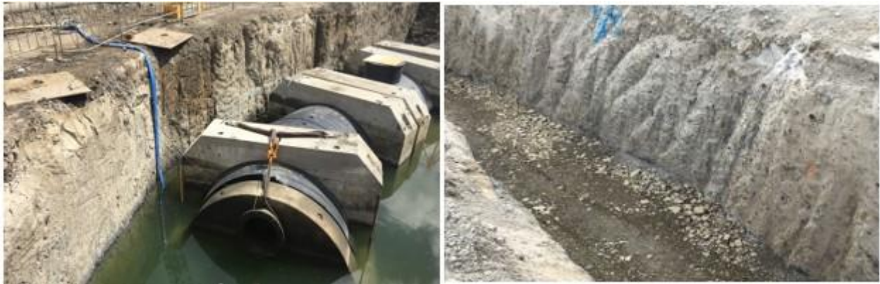
Figure 11: Open face of CSM wall
