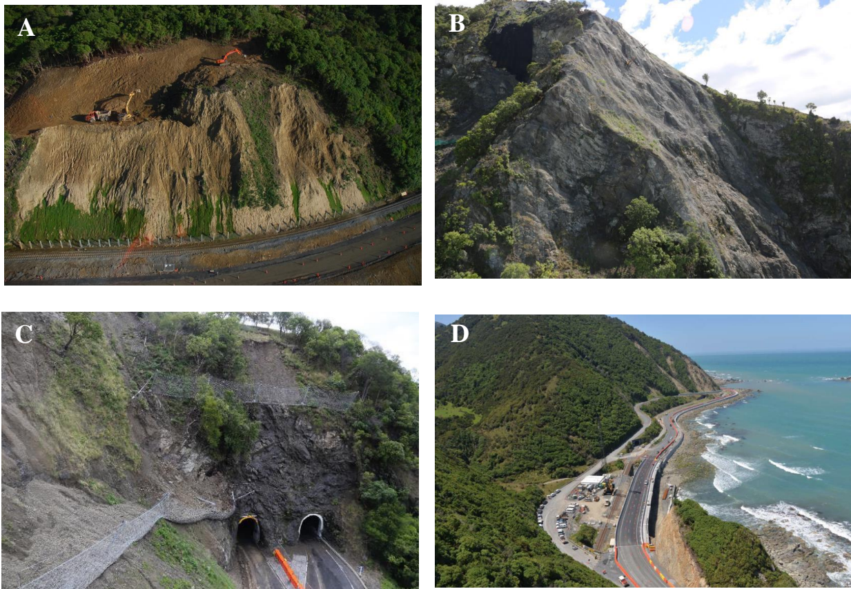
Figure 5: Examples of NCTIR recovery works. (A) Slope re-profiling and bulk earthworks. (B) Anchored rock fall netting. (C) Rock fall fences. (D) Realignment of the transport corridor.
