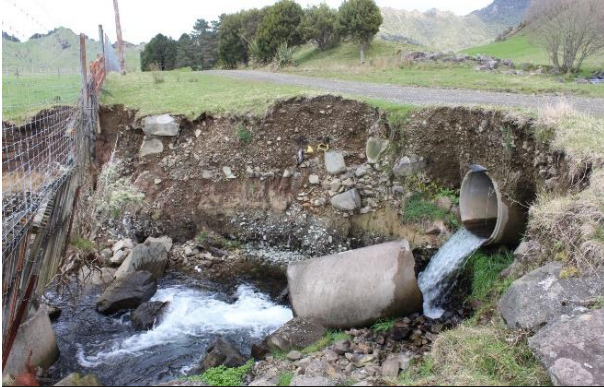
Culvert outlet scour at Moutohora Road, Motu
