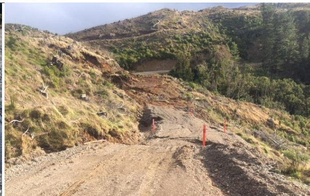
Hillside failure at Waitahaia Road, Te Puia Springs
