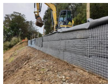
MSE wall at Arakihi Road RP 0.125
