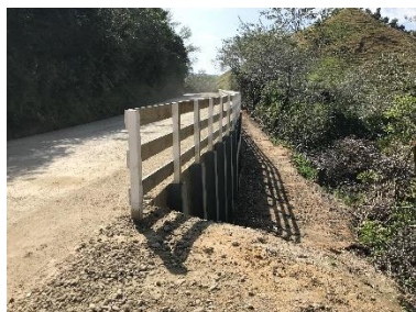
Timber retaining wall at Armstrong Road RP 2.557
