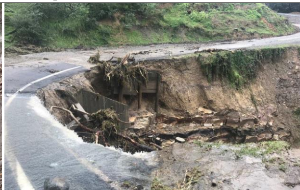
Scour due to culvert blockage and storm water runoff at Arakihi Road, Tolaga
