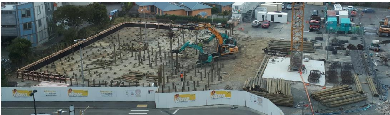
Figure 2: Timber pile installation
