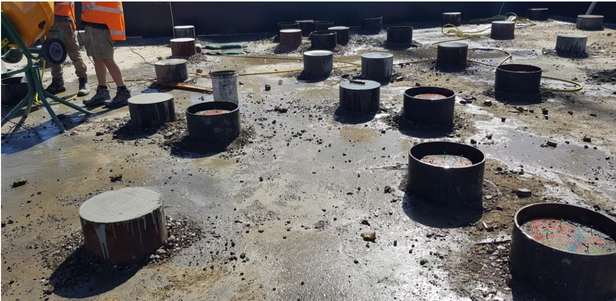
Figure 2: Pile caps undergoing grouting. Site level raised to top of pile caps with hardfill.
