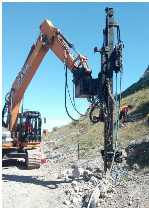
Figure 6: Excavator mounted drill rig installing self-drilling foundation micro-piles at Ohau Point
