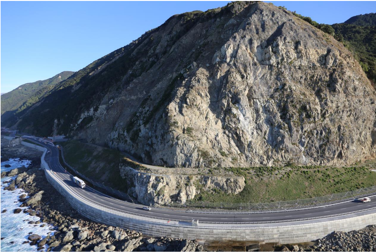
Figure 11: Ohau Point with the completed rockfall mitigation works in place.
