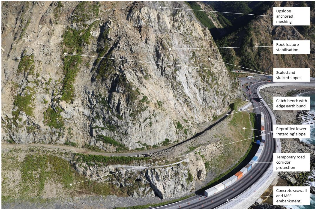
Figure 2: Works completed prior to commencement of 2000kJ barrier construction (Dec 2018)
