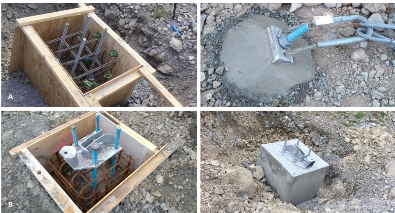
Figure 7 Plinth construction, note the variable particle sizes in the excavations. A) Landslide debris plinth detail B) Rock plinth detail C) Poured plinth awaiting backfill D) Bracing anchor flexed plinth detail.
