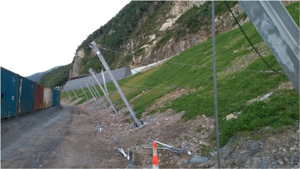
Figure 8: Partially constructed barrier, posts, foundations and bracing cables in place
