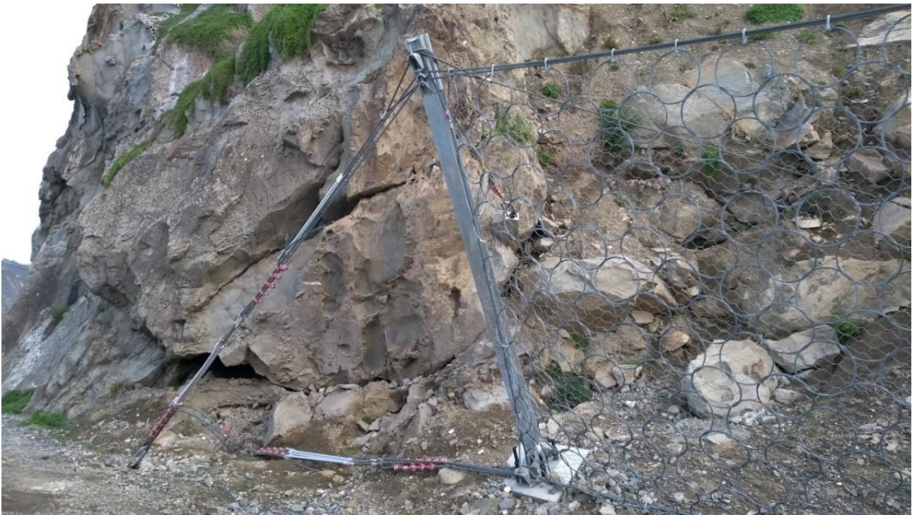
Figure 9 Southern end of 2000kJ B2 segment with modified upslope bracing cable geometry
