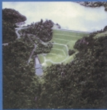
Feasibility, investigation, detail design Cosseys Dam upgrade, Hunua Ranges
