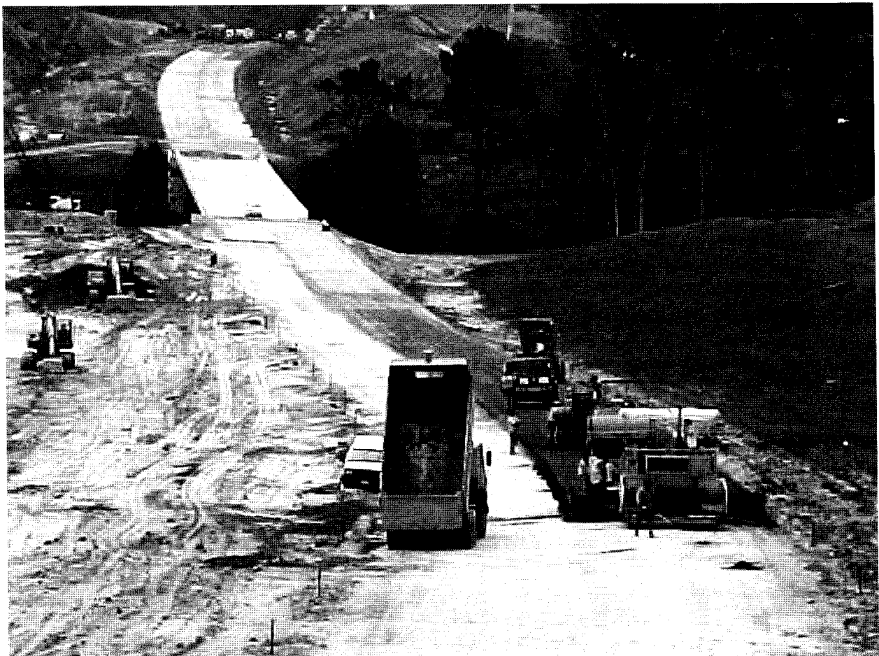
Looking North over Orewa South River Bridge
