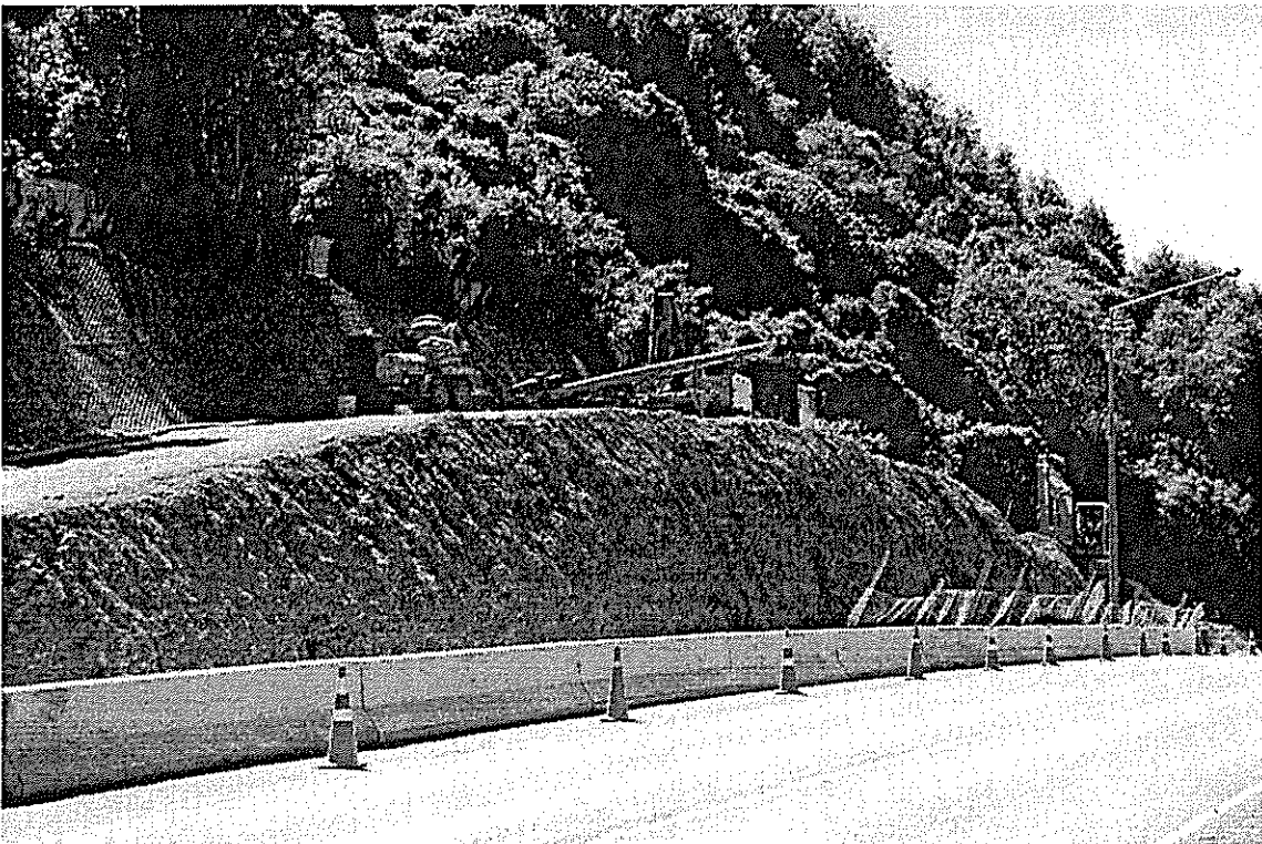
Figure 2 - Drilling rig installing soil nails and wire mesh on face.
