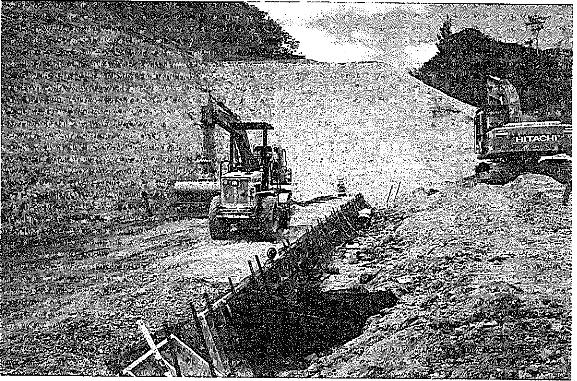
Photograph 1: Mohaka Hill, lower excavation and beginning reinforced slope
