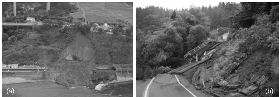
Figure 3: Examples of slope failures during the earthquake: (a) near JR Omigawa station (photo by Kokusai Kogyo Co. Ltd); and (b) along National Route No. 8 in Senbon, Nagaoka City (photo by Prof. Inoue).
